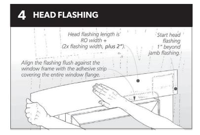
Wipe the head flange, jamb flashing and sheating with a clean rag. Cut the head flashing to twice the width of the rough opening + 2x the width of the flashing plus 2". Install the head flashing by pressing firmly in place in one direction to prevent voids.
